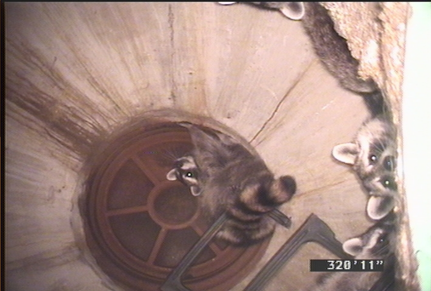
Raccoons Living in Manhole
